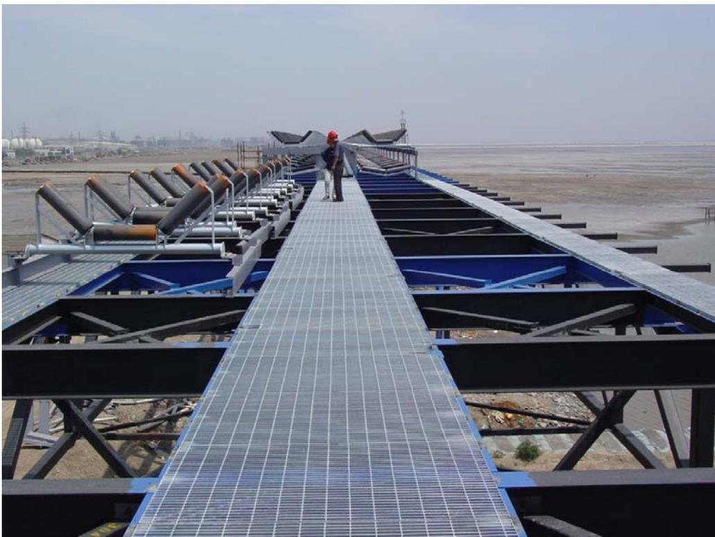
Figure 5. Tianjin Port Coal Conveyor Under Construction
